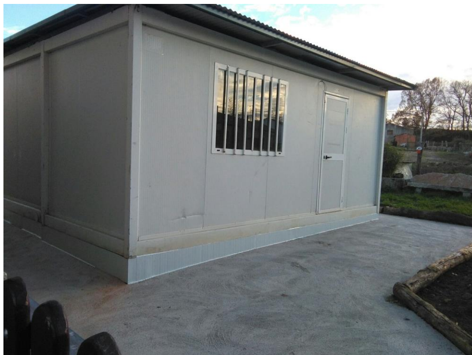
Prefabricated building – an innovative approach to starting a low-cost micro cheese dairy
